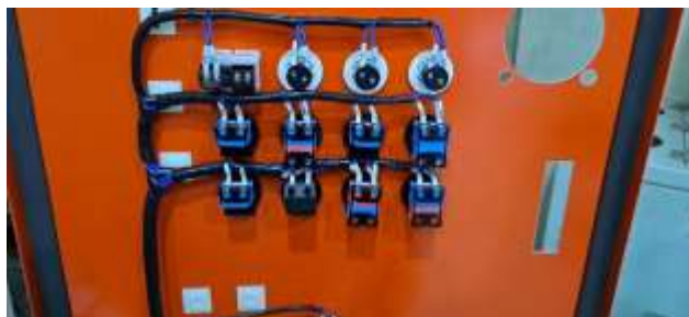
Gambar 2. 12 Wiring dan wrapping spiral panel mc water cooling supply
