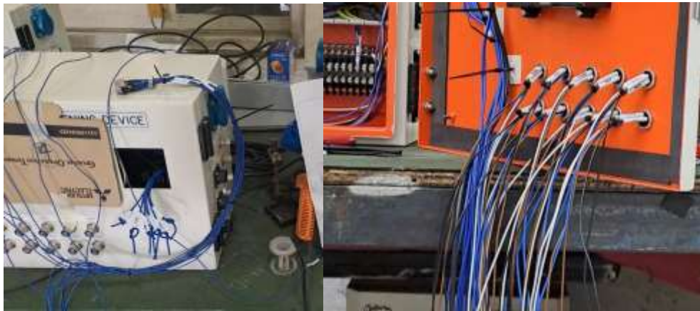
Gambar 2. 1 Penyolderan kabel panel Pokayoke Tightening Device
