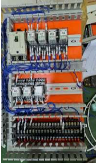
Gambar 2. 9 Wiring panel Quenching Tank Diasil BC
