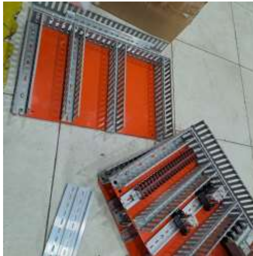
Gambar 2. 15 Pembuatan base plate panel P-Auto On/Off Electrical & Comp.
