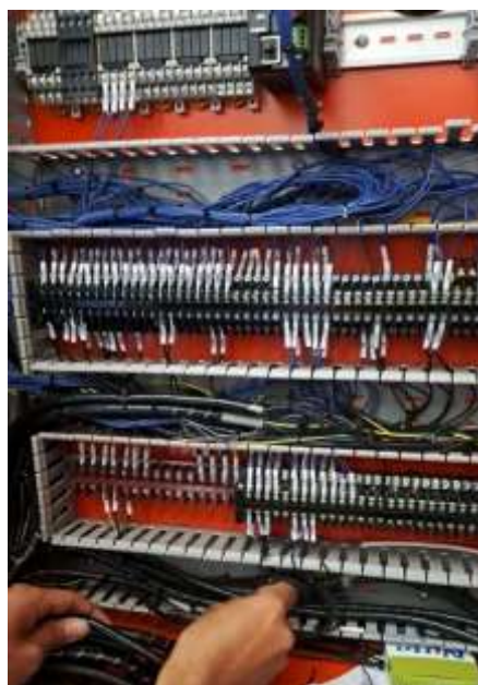
Gambar 2. 6 Wiring panel Crank Case EG Numbering MC
