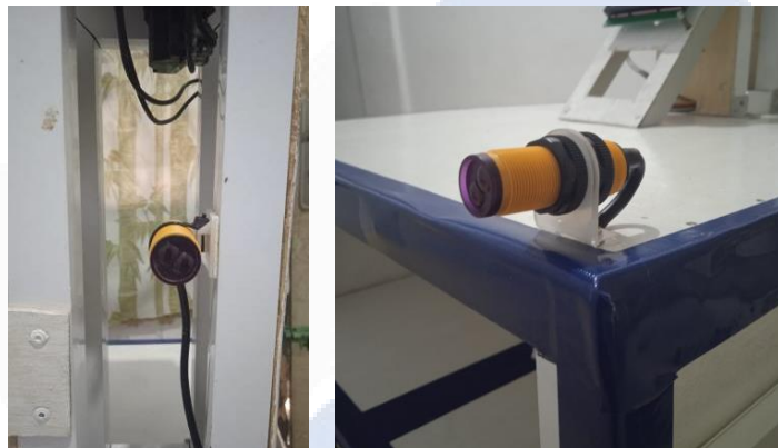
Gambar 4.4 Pemasangan Sensor Proximity
