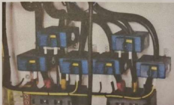
Gambar 2. 17 Sensor Current Trafo
