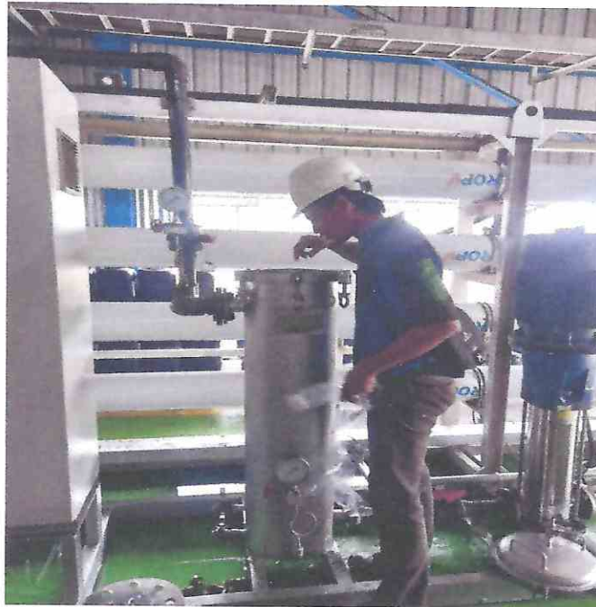
Gambar 2.6 Kegiatan pergantian filter air.
