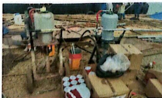
Gambar 1. 9 Blasting and Painting Equipment
