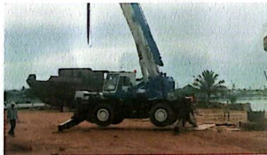
Gambar 1. 6 Rough Terrain Crane
