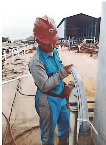
Gambar 2.17 Pengisian air tangki ballast.
