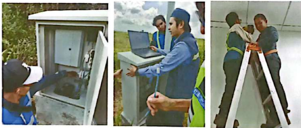
Gambar 18. Proses Pengecekan Panel CCTV dan Maintenance CCTV
