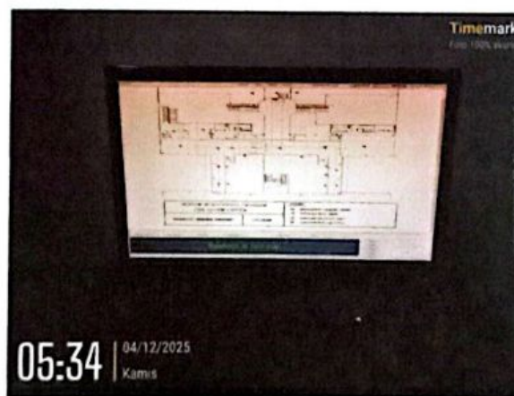
Gambar 14. Main Control Fire Alarm (MCFA)
