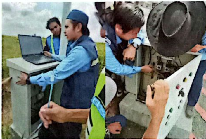
Gambar 18. Proses Pengecekan Panel CCTV dan Maintenance CCTV
