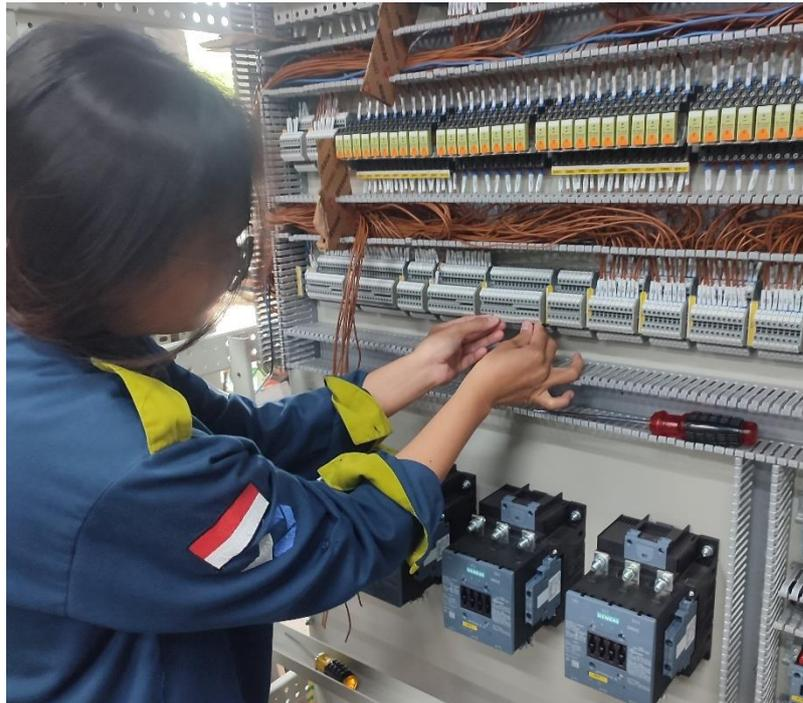
Gambar 2. 5 *Marking* komponen PANEL COS CMP VSD Cell 1
