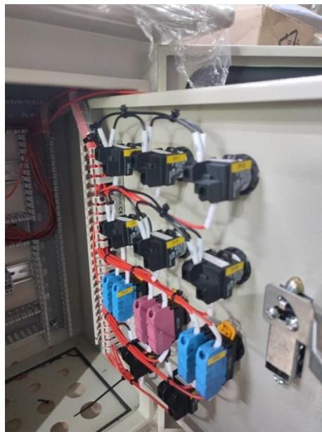
Gambar 2. 24 *Wiring* Komponen PANEL LCS *SECONDARY CRUSHER A*
