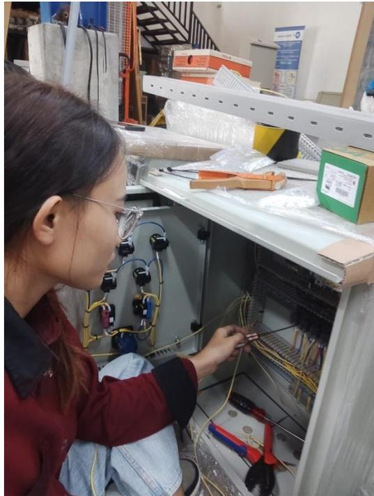
Gambar 2. 29 *Wiring Relay PANEL DOL FOR PUMP*
