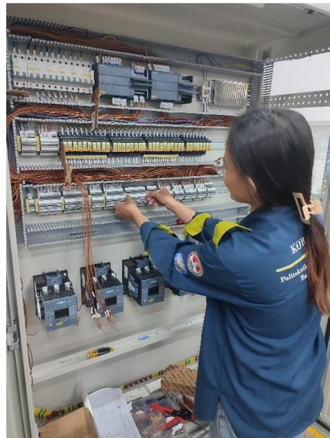
Gambar 2. 8 *Wiring relay PANEL COS CMP VSD Cell 3*
