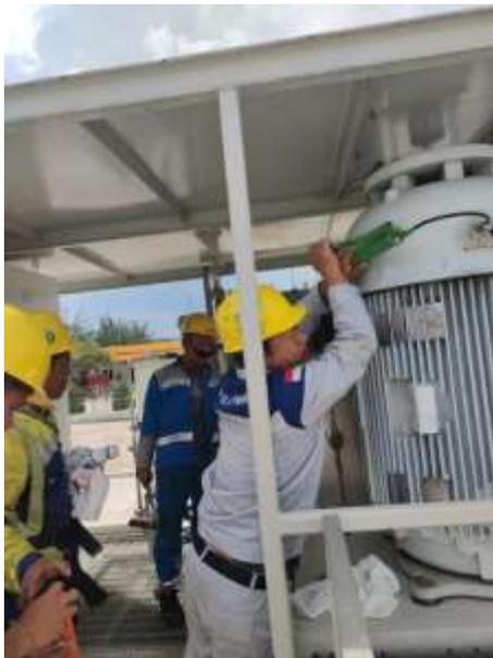
2.1. *Grease Bearing motor*
