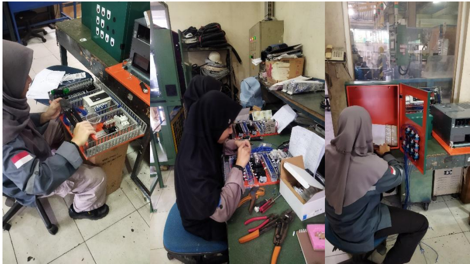
Gambar 2. 1 Proses Wiring Panel
