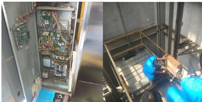
Gambar 10 Panel Sistem Kontrol Lift
