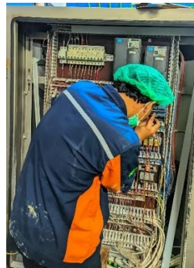
Gambar 2. 22 Wiring Modul PLC PT MACHROPRIMA PANGANUTAMA
