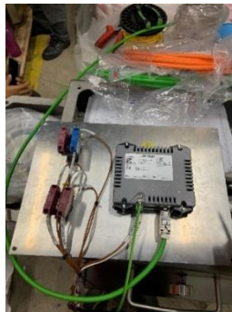
Gambar 2. 10 Terminasi Kabel HMI, Emergency, Selector Switch PT.Machroprima Panganutama
