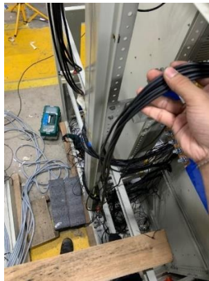
Gambar 2. 6 Terminasi Outgoing Star Delta PT.ATMINDO
