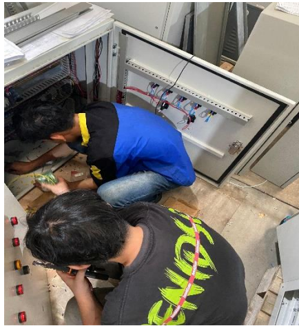
Gambar 2.7 Proses Wiring Panel
