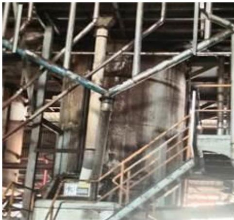
*Gambar 2.8 Sand Trap Tank*
