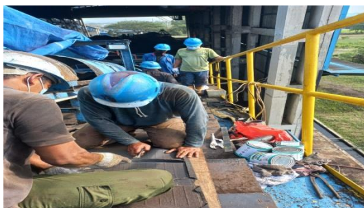
Gambar 2.12 Pengupasan belt Panjang Pengupasan belt 65cm Kemiringan pengupasan belt 15°
