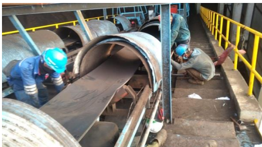
Gambar 2.16 Penaikan belt ke conveyor 2A
