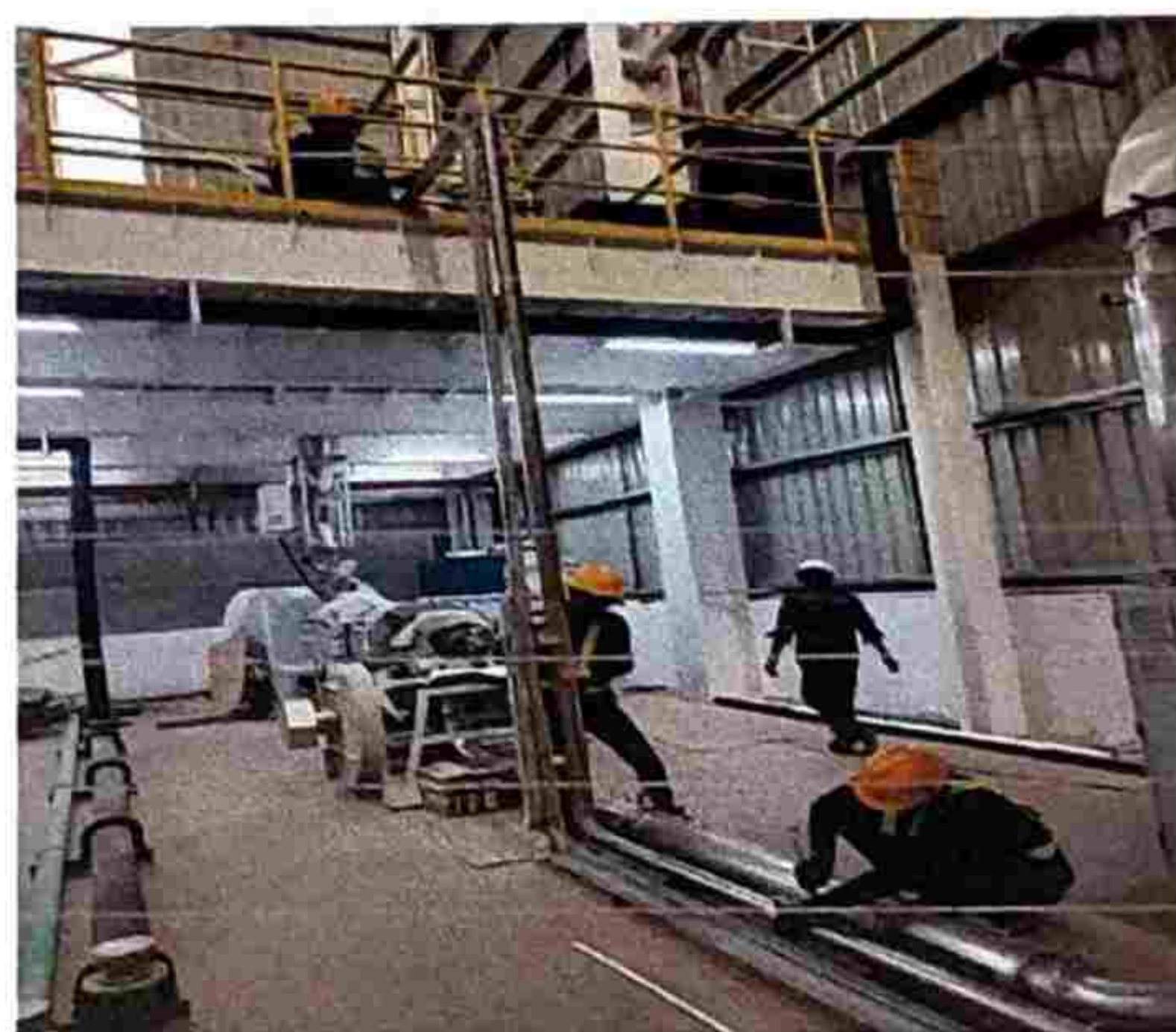
Gambar 2. 11 Installation Stainles Pipe Machine Pallettaizer
