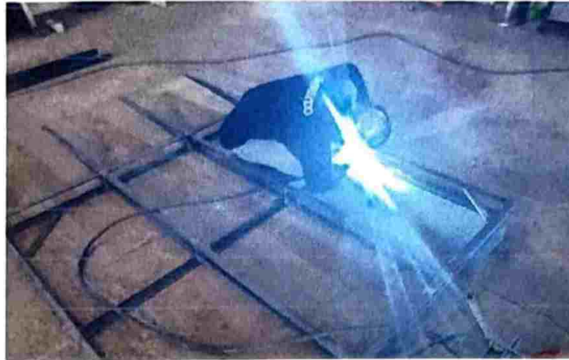
Gambar 2. 4 Fabrication Deck Top Coat
