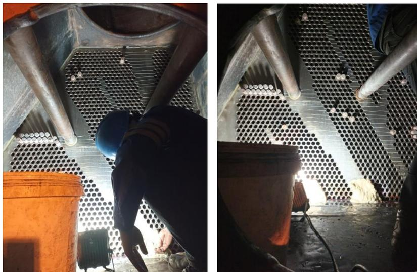
Gambar 2.5 *Tube* Kondensor
