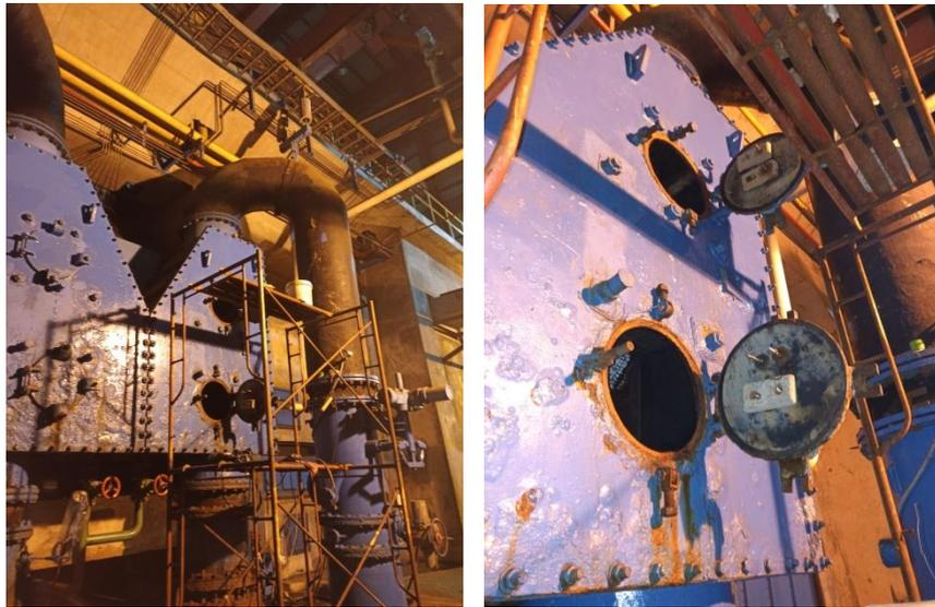
Gambar 2.4 *Main Hole* Kondensor
