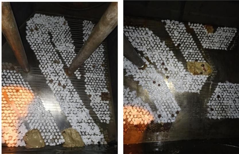
Gambar 2.6 *Tube* Kondensor
