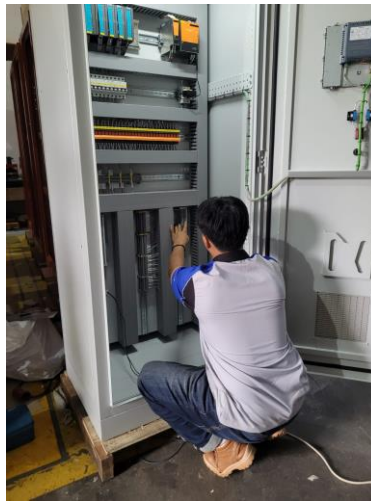
Gambar 2.15 Wiring panel
