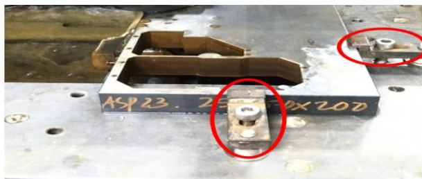
Gambar 2.7 Proses setting material
