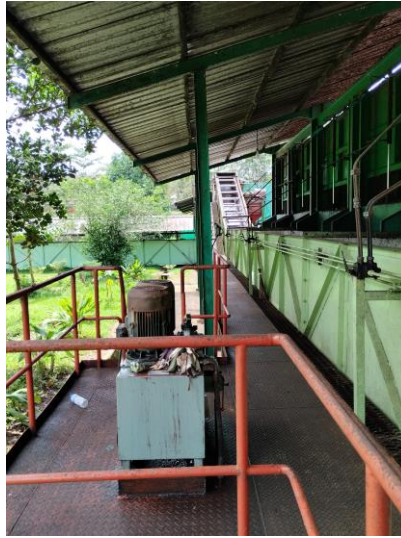
Gambar 2.3 Station Loading Ramp
