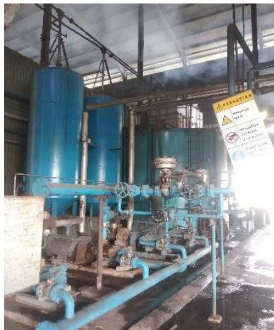
Gambar 2. 21 Softener Tank
