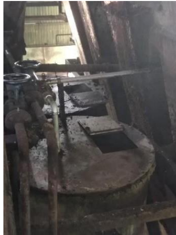
Gambar 2. 11 Sand Trap Tank
