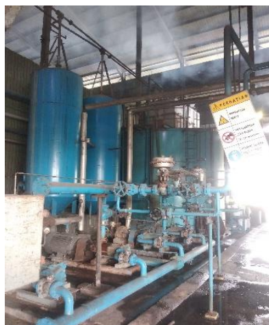
Gambar 2. 21 Softener Tank
