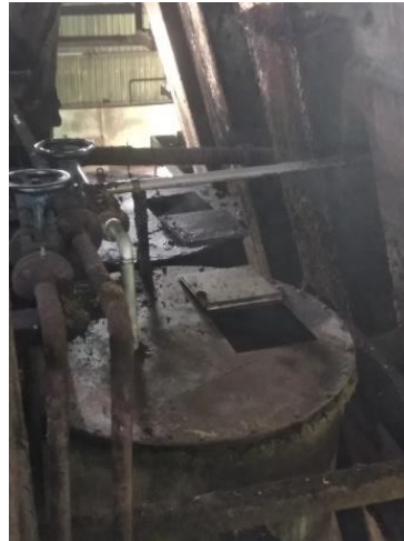
Gambar 2. 11 Sand Trap Tank
