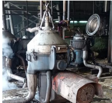
Gambar 2. 14 Sparator
