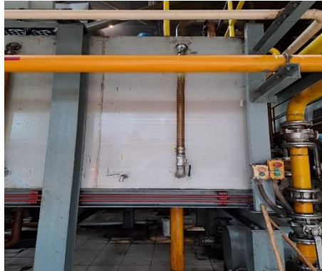
Gambar 1. 27 Clean Oil Tank
