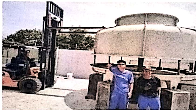
Gambar 1.18 pemasangan colling tower
