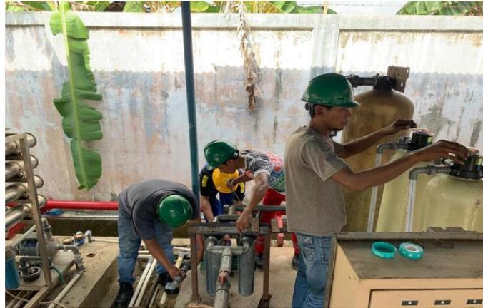
Gambar 2.3 install water softener
