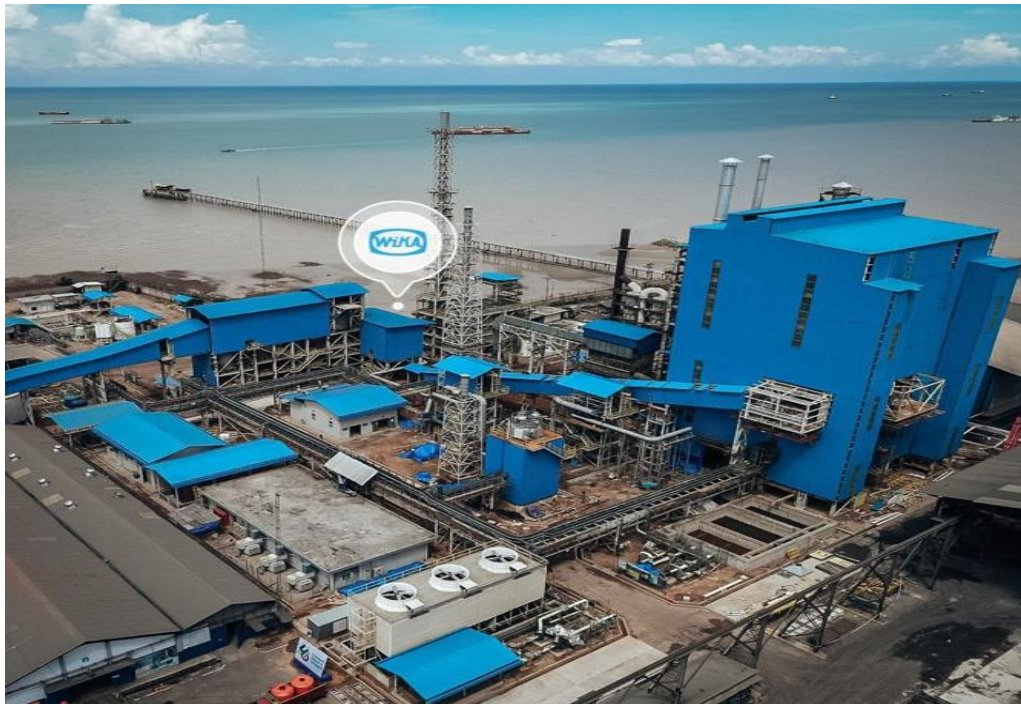
Gambar 1.2 Proyek EPCC TSL AUSMELT FURNACE PT. TIMAH Tbk
