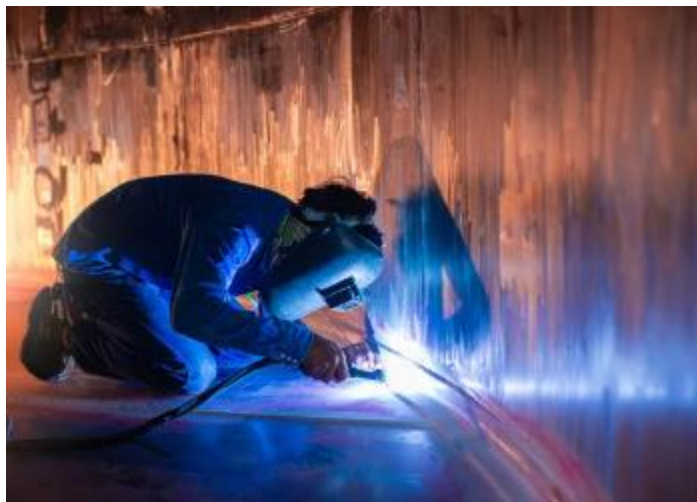
Gambar 2.3 Pengelasan Joint Plate Tank
