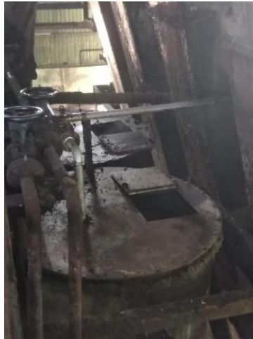
Gambar 2. 11 Sand Trap Tank
