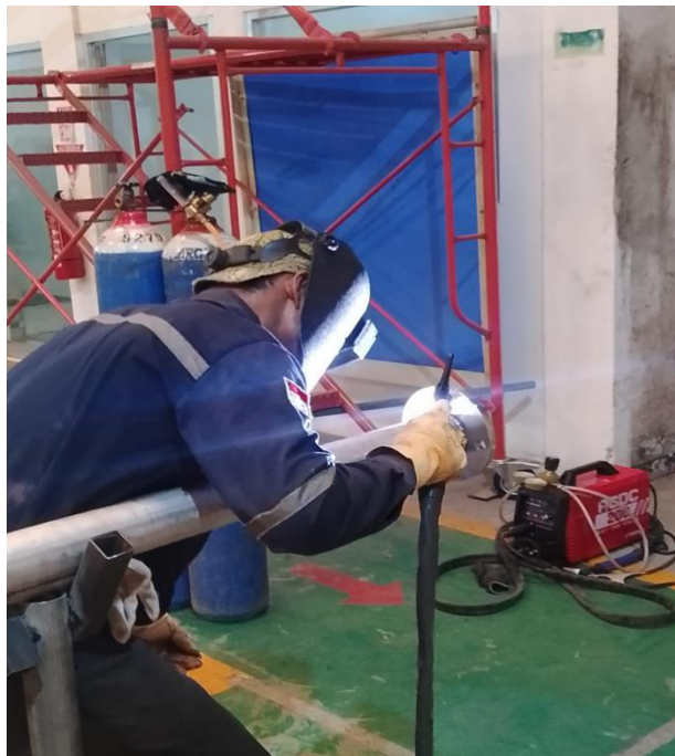
Gambar 2.6 Fabrication Stainless Pipe.
