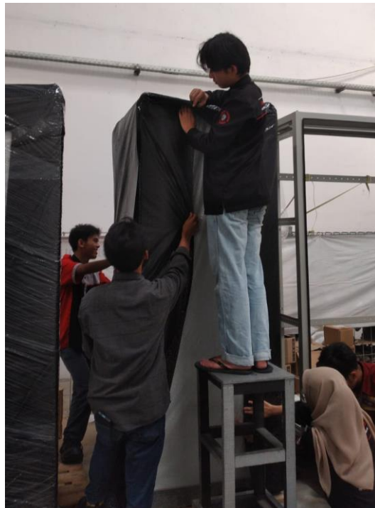
Gambar 2. 8 Pemasangan Bubble Wrap Panel SDP Utility 4
