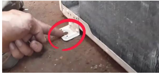
Gambar 4.13 memasang bracket outdoor
