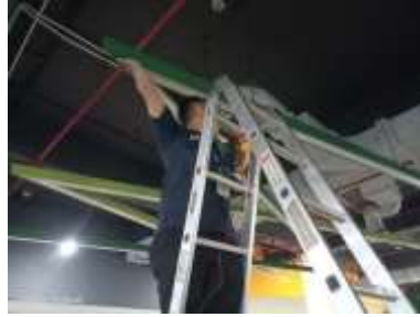
Gambar 2.34 Servis Bulanan FCU Ducting
