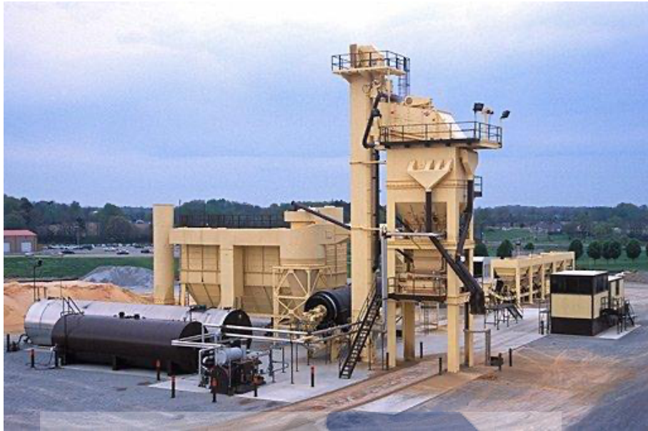
(Gambar 2.3 Asphalt mixing plant)
