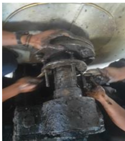
Gambar 2. 3 Penggantian Paking Auger Sterilizer
