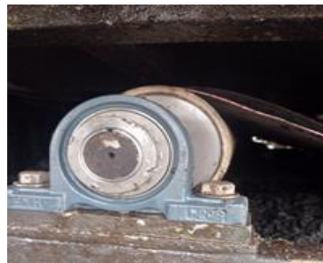
Gambar 2. 13 Penggantian Bearing Mesin Belt Press
