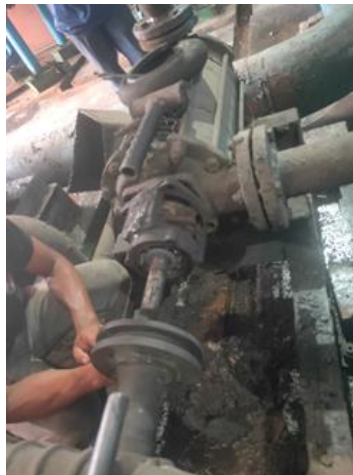
Gambar 2. 11 Perbaikan Pompa Feed Pump Boiler
