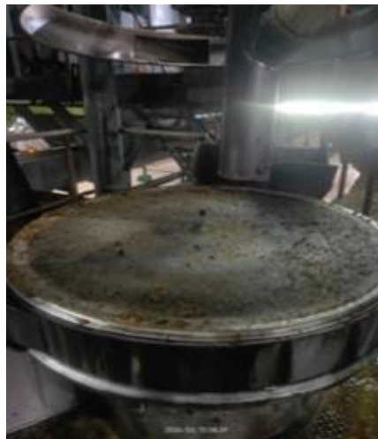
Gambar 2. 9 Perbaikan Vibrating Screen Clarification
