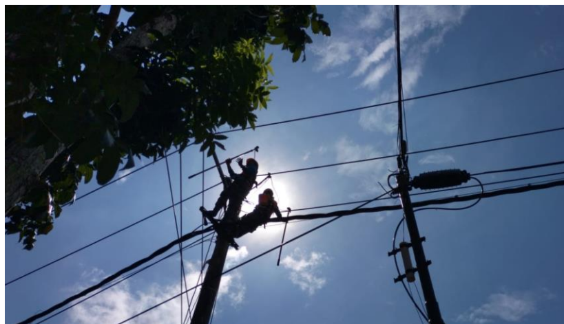
Gambar 2.37 Proses pasang ground
