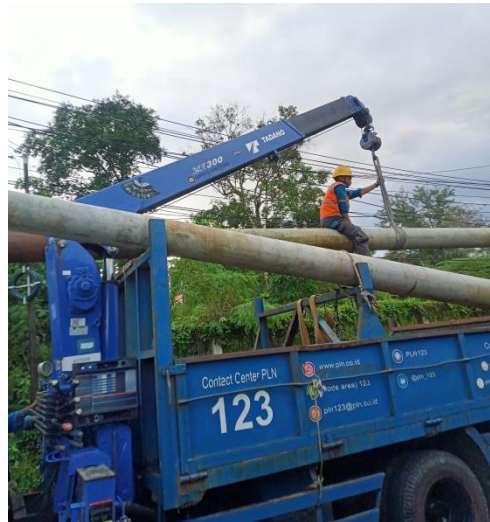
Gambar 2.32 Proses cabut tiang beton gardu distribusi
