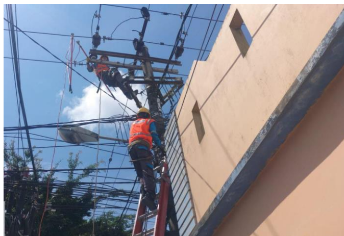
Gambar 2.33 Proses pasang ground
