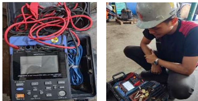
Gambar 2.1 Proses Pengecekan Insulation Megger Test
