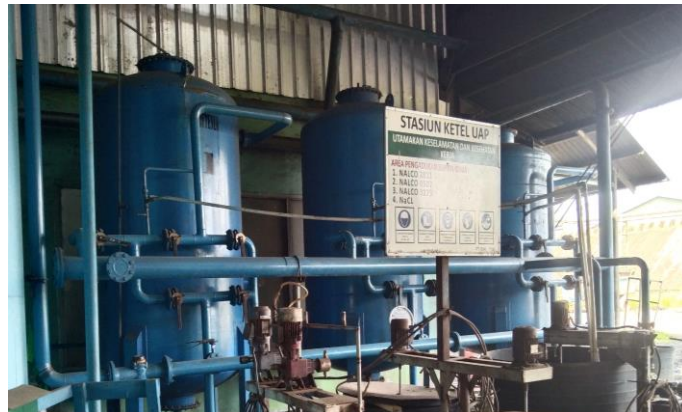
Gambar 2.23 Softener Tank
