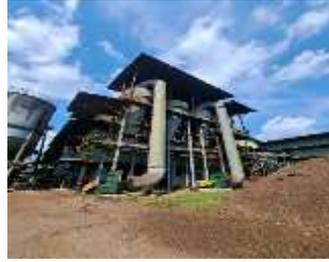
Gambar 2.14 Fibre Cyclone
