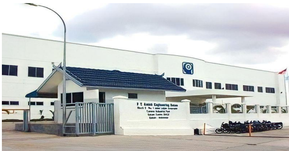
Gambar 1.1 PT. Ennovi Engineering Batam
