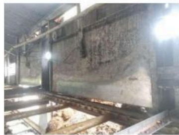
Gambar 2.1. Pintu loading ramp
