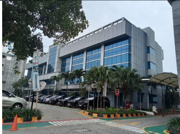
Gambar 1.1. 3 Kantor Tampak Samping
