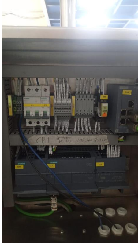
Gambar 2. 27 Hasil pengerjaan wiring PLC panel Weighing Table PT. Natural Indococonut
