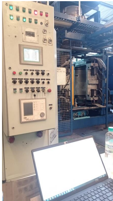
Gambar 2. 20 Proses Troubleshooting Modifikasi Program di PT. Novo Complast Indonesia
