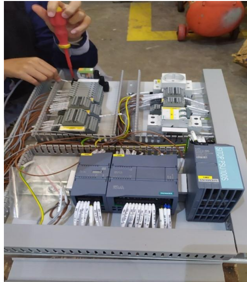
Gambar 2. 5 Wiring Panel Husky PSD dan National Office PT. Coca Cola Bottling Indonesia
