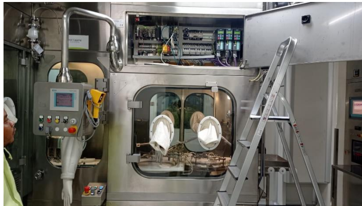
Gambar 2. 17 Pengerjaan pergantian VSD motor di PT. Fonko International Pharmaceuticals
