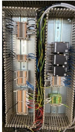
Gambar 2. 21 Wiring Panel JB
