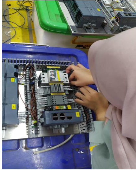
Gambar 2. 23 Proses Wiring PLC Panel Weighing Table
