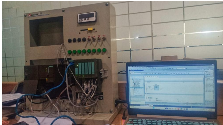
Gambar 2. 2 Training PLC SIEMENS
