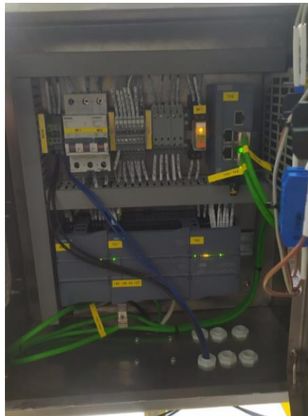
Gambar 2. 24 Hasil Wiring PLC Panel Weighing Table
