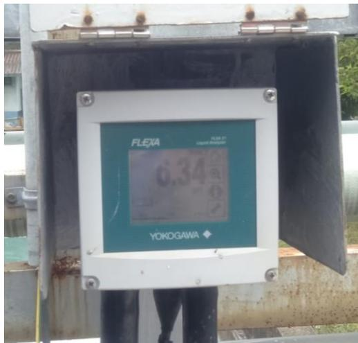
*Gambar 2. 2 Monitoring Nilai Ph Air di WTP(Water Treatment Plane)*
