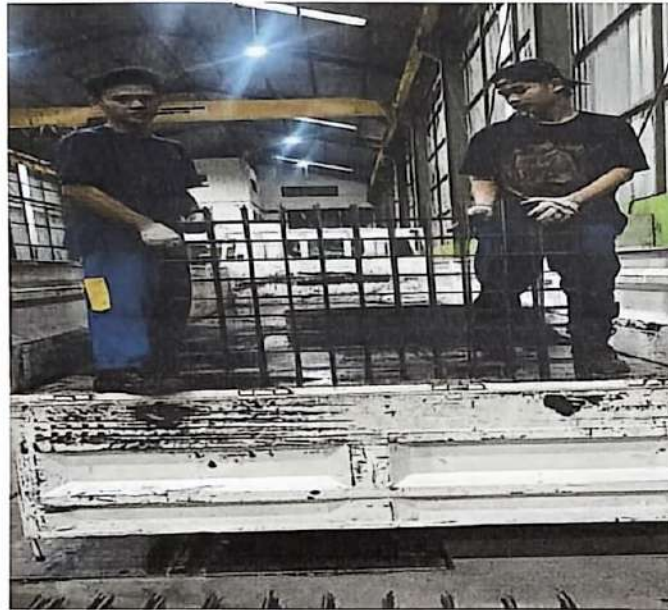
Gambar 2.4 Proses Bongkar Wiremesh
