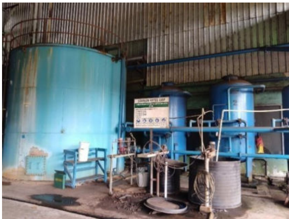
Gambar 2.24 Softener Tank
