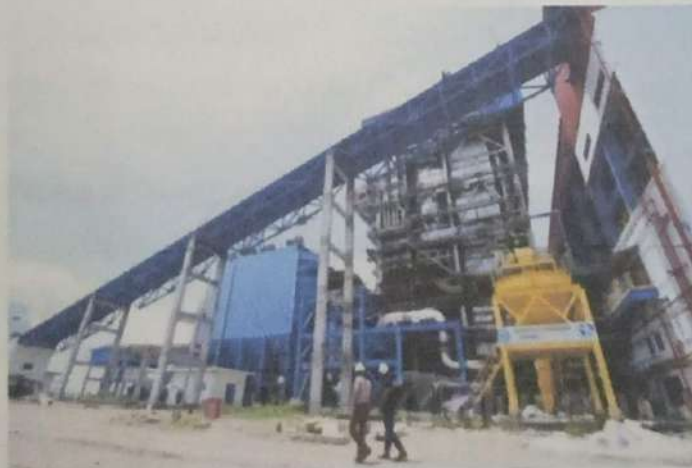
Gambar 1 1.1 PT PJB Services Unit 3 PLTU Bangka
