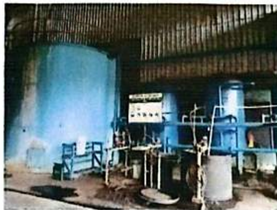
Gambar 2.24 Softener Tank
