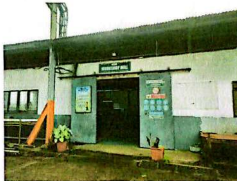
Gambar 2. 1 Workshop Mill PT. Steelindo Wahana Perkasa
